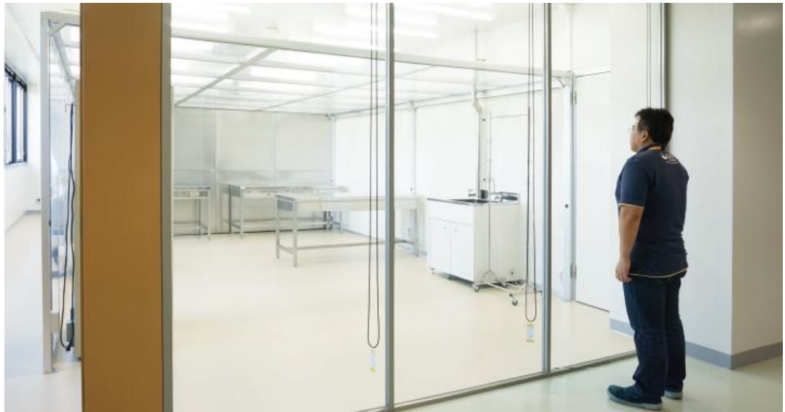
Floor KOACH installed on the third floor of the Kochi Institute for Core Sample Research (Photo from the December 2015 issue of this CHS News).
